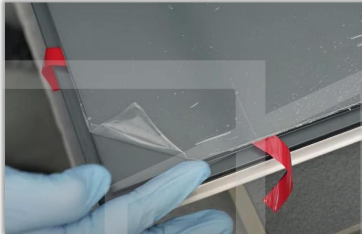
5. Remove the red release paper by pulling the sections previously folded out.
