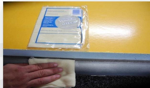
Then, using the SIKA POWER CLEAN AID sponge and the SIKA AKTIVATOR PRO agent, wipe the surface of the leaf and the metal sheet at the gluing location.
