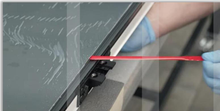
6. Set and press the panel onto the door leaf, and the metal sheet panels are immobilised by the tape. The use a roller is recommended.
