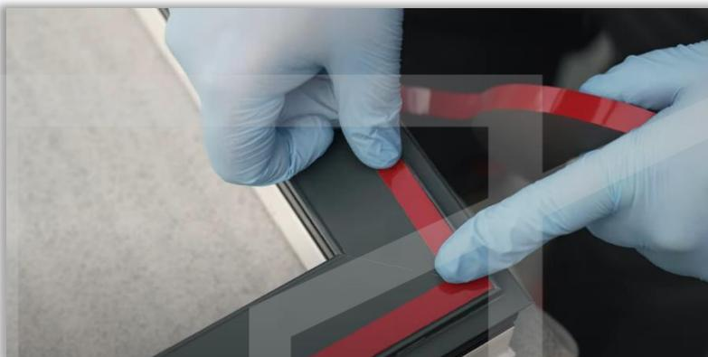
2. Apply the Sikaflex 221 glue (according to the recommendations in the instruction, **section 3 "Gluing"**).
